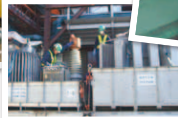
Removal of transformers containing PCBs/Inazawa Plant
